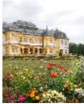
Vh.I, Westfassade, DI014645, BSV-
