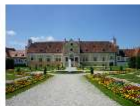
SAS.I, West-Fassade, DI009737, BSV
