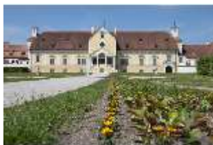
SAS.I, Ostfassade, DI014465, BSV
