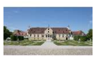
SAS.I, Ostfassade, DI014464, BSV
