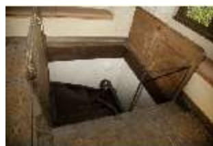
Ro.II, Casino, Turmzimmer, Treppe, DI002745, BSV
