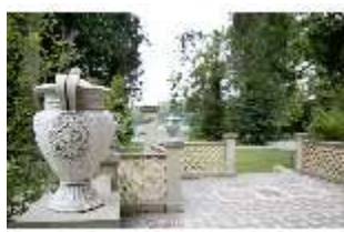
Ro.I, Casino, große Terrasse, Vase, Balustrade, DI006650, BSV
