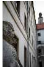
ND.I, Innenhof, Ostfassade, DI027419, BSV
