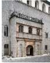
ND.I, Portalaltane, westl. Fassade, DE001382, BSV
