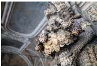
ResMü.II, Detail, Felsenbrunnenanlage, Grottenhof, R. 6, DI028786, RSV-
