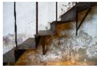
HchAS.II, Inseldom, Treppe, DI038653, BSV-
