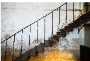
HchAS.II, Inseldom, Treppe, DI038650, BSV-
