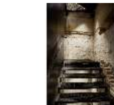
HchAS.II, Inseldom, Treppe, DI020322, BSV
