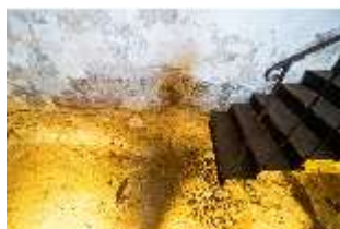
HchAS.II, Inseldom, Treppe, DI038651, BSV-
