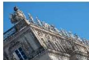
HchNS.I, Westfassade (Detail), DI018946, BSV
