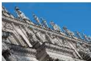
HchNS.I, Westfassade (Detail), DI018949, BSV
