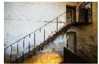
HchAS.II, Inseldom, Treppe, DI038649, BSV-
