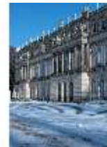
HchNS.I, Westfassade (Detail), DI018947, BSV
