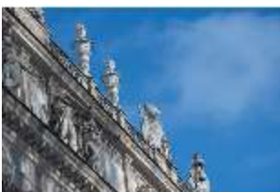
HchNS.I, Westfassade (Detail), DI018948, BSV
