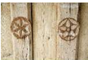
Pr.II, Holzdecke, Detail, R.2, DI001221, BSV
