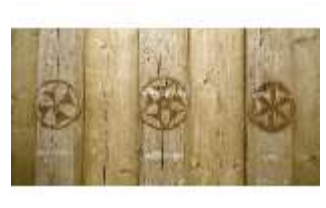
Pr.II, Holzdecke, Detail, R.2, DI001220, BSV
