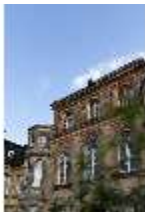
BayFa.I, Nordfassade (Detail), DI017166, BSV-
