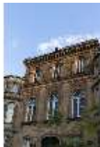
BayFa.I, Nordfassade (Detail), DI017167, BSV-
