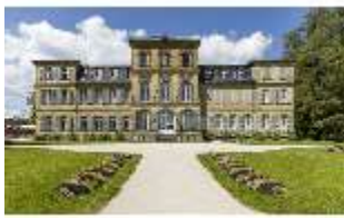
BayFa.I, Südfassade, DI002641, BSV
