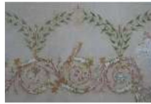
AschPomp.II, Loggia, Detail oberes Wandfries, DI013973, BSV-
