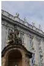
AnsRes.I, Residenz, Hauptfass. m. Wachhs./ Schilderhs., DI024128, BSV-
